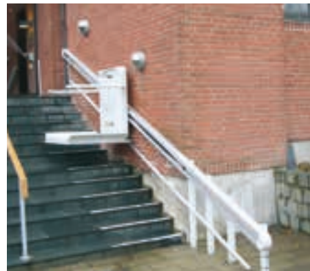
Outdoor installation: partly wall, partly stanchions. Church, Denmark.
