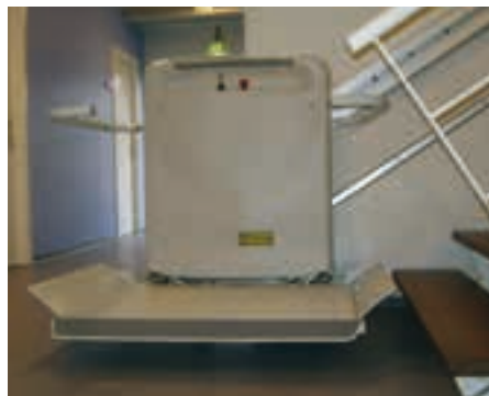
Indoor installation in a walk through hall limiting free space down stairs. After use lift will be folded up and drive up the stairs to be parked away.
