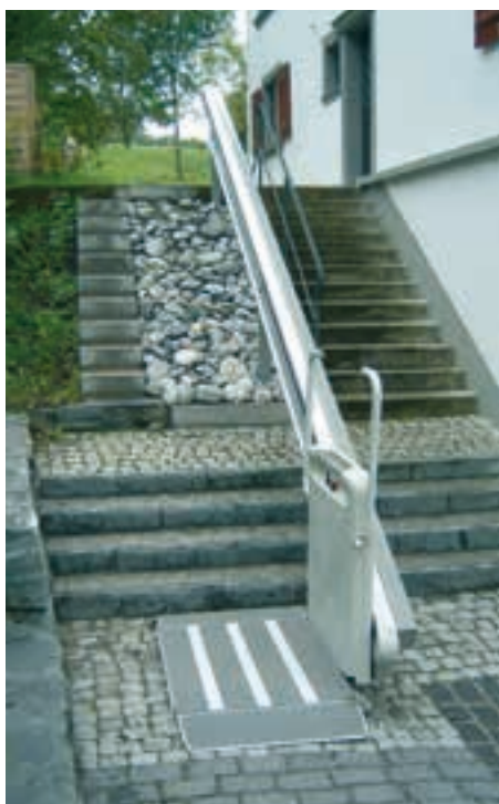
Outdoor installation. Slides down slope next to stairs. Private home, Switzerland.
