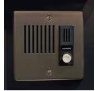
Aiphone interphone Connects the caller to an internal front desk or similar.
